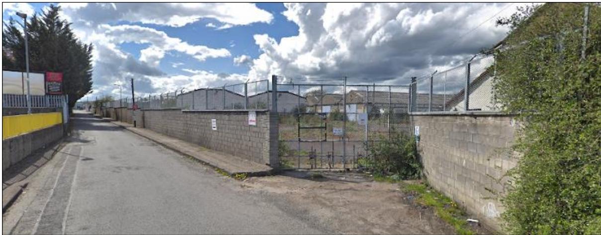
Figure 5.0 Image of the subject site as viewed from the estate road abutting the site's southern boundary looking north-west
